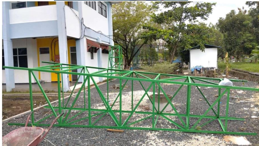
Gambar 5.5 Proses pengecatan
